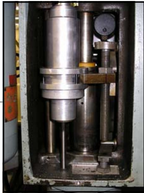
Before —with Drill Demon 4002-31-x installed.
